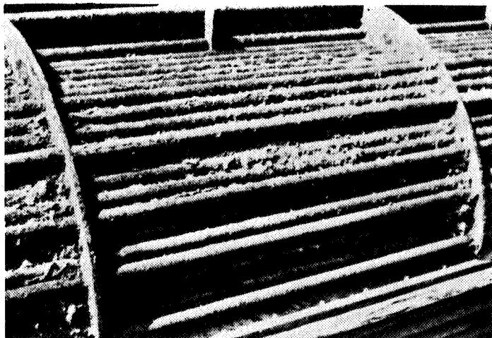
Figure 7. Photo of syn gas intercooler bundle pulled in February, 1973.
